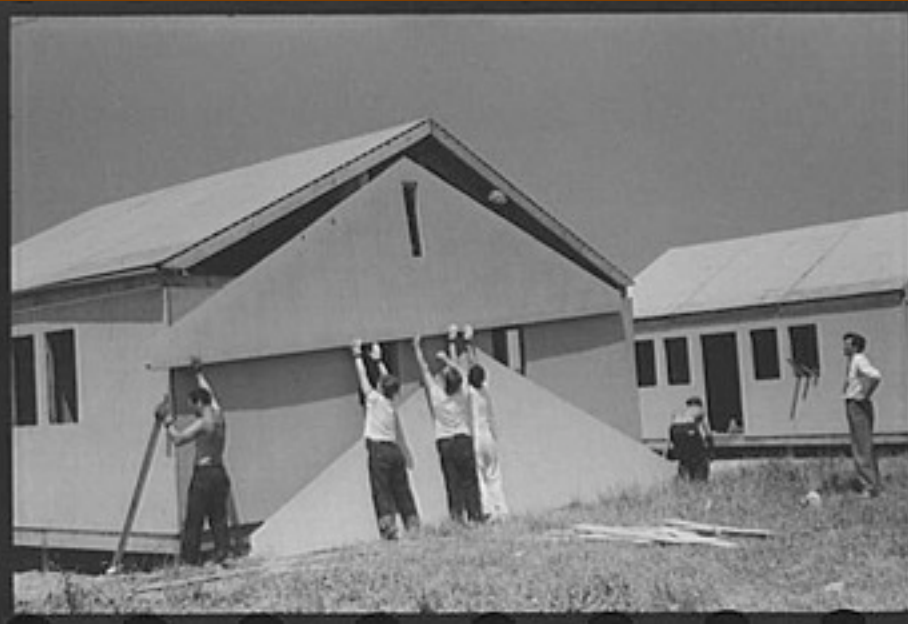
PWA workers construct a public building in Hartford, Connecticut
