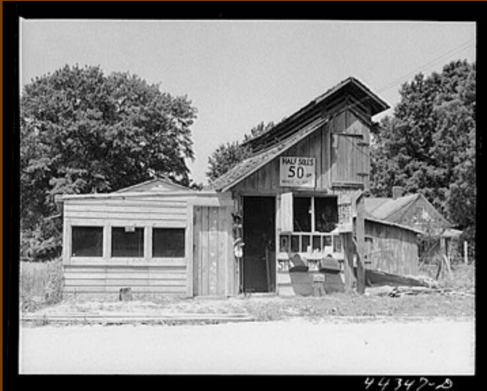
Repaired business in Childersburg, Alabama
